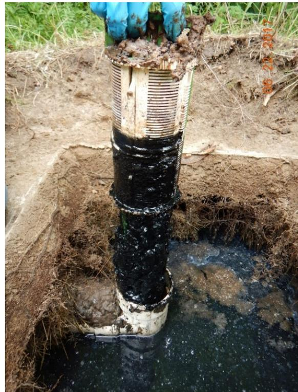
**Figure 2. Dirty effluent filter requiring remedial action [Photo credit: Mississippi Rideau Septic System Office]**
